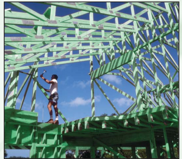
The FrameGuard® coating keeps lumber looking cleaner and brighter during storage, construction, and beyond. This is especially important to truss and component manufacturers whose end products tend to be exposed to the elements longer than other framing materials.
