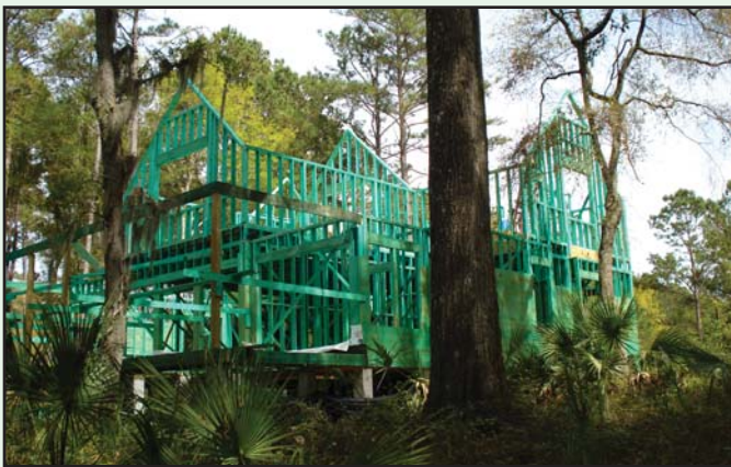
FrameGuard® wood protects this South Carolina home from mold, termites, and fungal decay.
