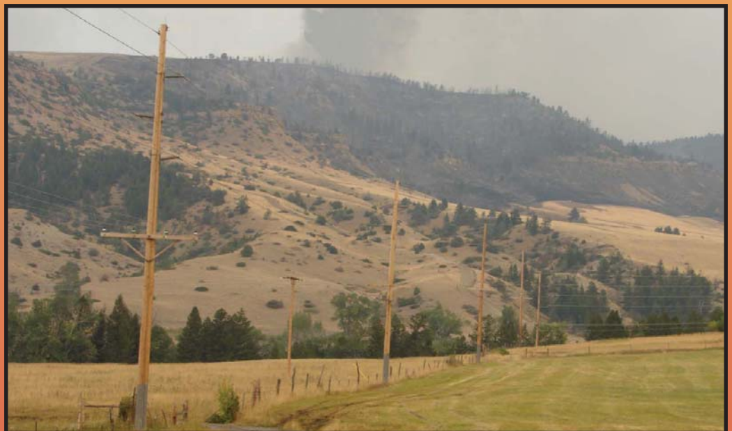
At right is a line of poles treated with fire retardant coating; in the background, smoke appears from an approaching wildfire. Above is a coated pole and an uncoated pole after a field test.
