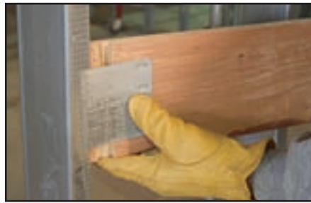
SNAP the Starter Edge into the open side of the stud flange
