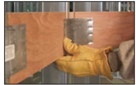
FLEX around stud flange using the flexible connector plate
