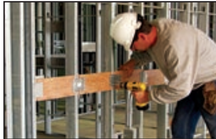
SCREW each plate to the stud flange using two small pan or wafer head screws
