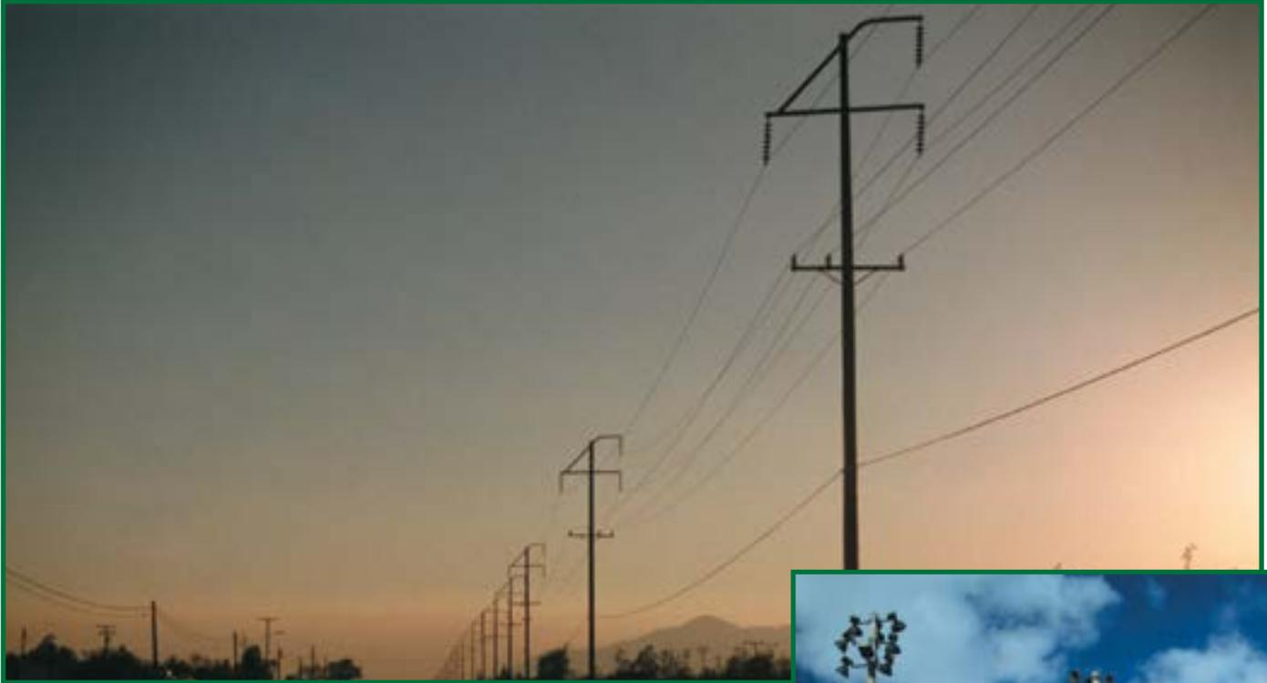
Warranted Chemonite® poles provide reliable transmission and distribution of electric energy, with practical benefits and less environmental impact than alternatives. The ACZA treatment consistently meets recognized standards of penetration and retention in difficult-to-treat species such as Douglas fir.
