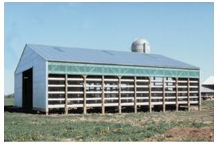
Wolmanized® CCA Heavy Duty $^{\text{m}}$  wood is an ideal structural material for today's farmers and ranchers in post frame construction as well as in the construction of pole barns.
