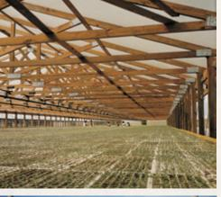
Wolmanized® CCA Heavy Duty™ wood combats the insect exposure and deterioration that occurs in barns and utility sheds.
