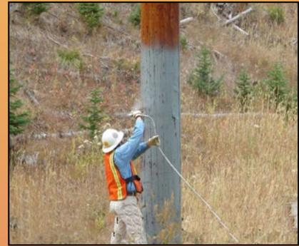
For typical grassland conditions, FireSheath™ coating is applied to a height of 6'. Here coating was spread to 10'. In dense forested areas or where brush is high, it may be advantageous to go higher.
