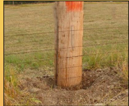
Shallow excavations were dug around each pole. A depth of only 1" to 2" is necessary; just enough to coat the groundline.
