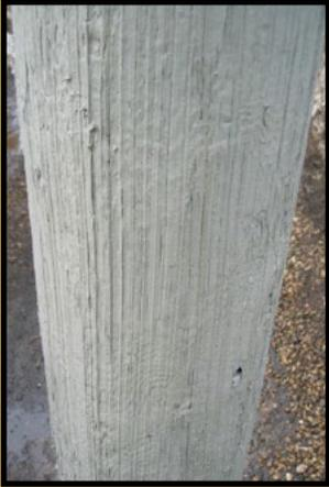
No longer does fire have to be a threat to your poles. A field-applied fire retardant coating called FireSheath™ fire retardant coating will help protect poles against the common types of fire that can damage or even topple a pole.
