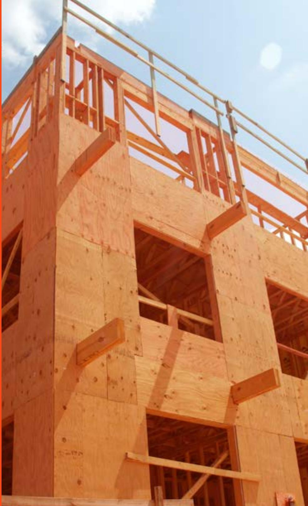
Since 1981, Dricon® fire retardant treated (FRT) wood has performed as intended in countless structures around the world, providing a convenient and economical building alternative. Pressure-treated for protection in the event of a fire, Dricon® FRT wood reduces flame spread and smoke development, the #1 killer in fires.
